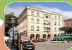
Municipal building Rathaus
