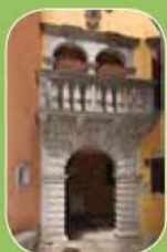
Franchovich palace Franchovich-Palast
